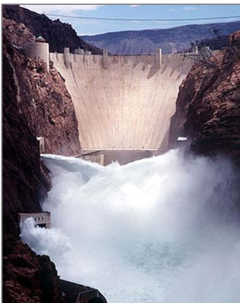
The Hoover Dam, the largest in the world at the time of its construction during the Great Depression, uses the power of the Colorado River to electrify the region.
