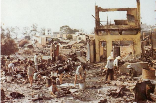
Civilians sort through the ruins of their homes in Cholon, the heavily damaged Chinese section of Saigon, after Tet Offensive operations in 1968.
