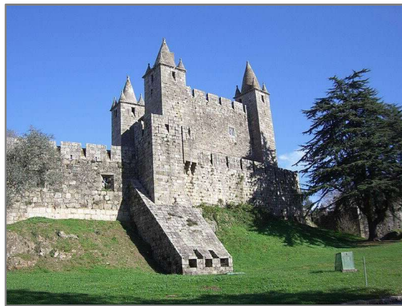
Santa Maria da Feira Castle in Portugal, with its 15 th century pinnacles
